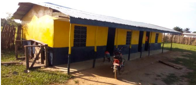
Anna E. Hall 3-classroom annex on March 16, 2023.
