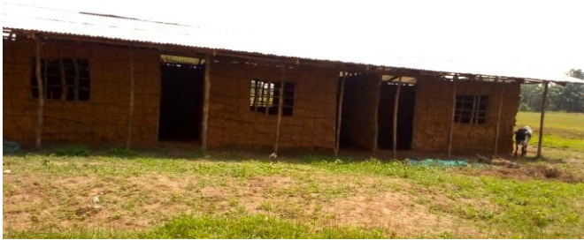
Anna E. Hall 3-classroom annex under construction on January 24, 2023.
